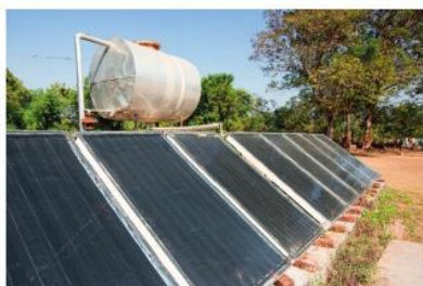
▲ Figure 17.14 Solar heating panels used to heat water
